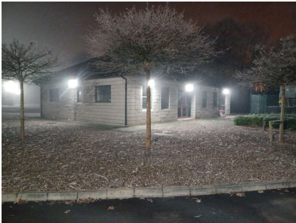
Figure 11-17: Existing Lighting on Buildings
