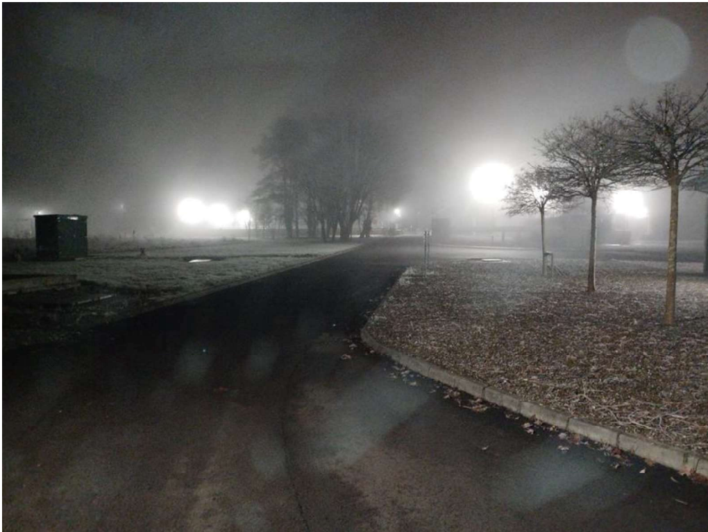
Figure 11-12: Current lighting situation at Castletroy WwTP
